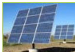
Solar system and equipment
